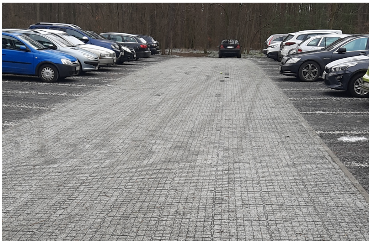
Figure 2. Example of rainwater permeable parking places and manoeuvring area—Zielona Góra, Cisowa Street.
