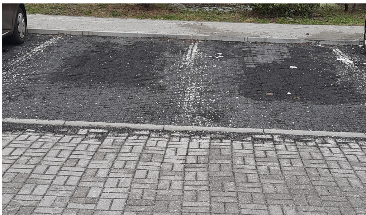
Figure 1. Example of rainwater permeable parking places—Zielona Góra, Cisowa Street.
